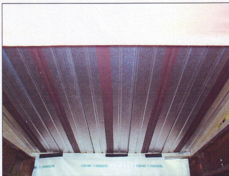
Figure 3 Dedpan® DS2020 RDV self-adhesive strips on underside centre of roofing bays
